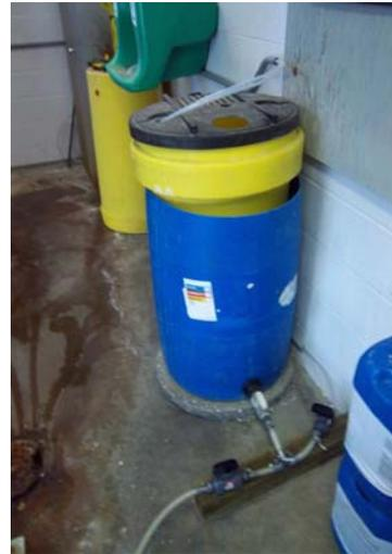
The Well #2 Chlorination System project was required by the State of Vermont through a 2011 Sanitary Survey. Well #2 is a backup water supply and is rarely used. The purpose of the project was to install a permanent stand-by chlorine feed system on the discharge piping of Well #2 to provide the capability for continuous disinfection.
