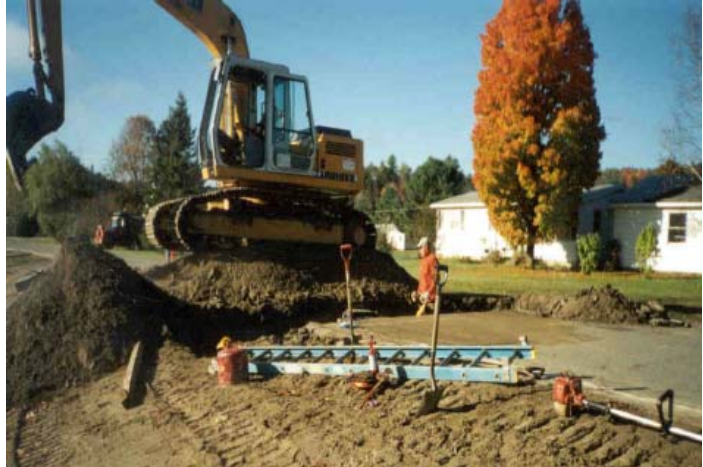
Heath Construction Begins Work in Early October
