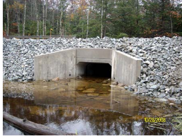
Replacement Box Culvert
