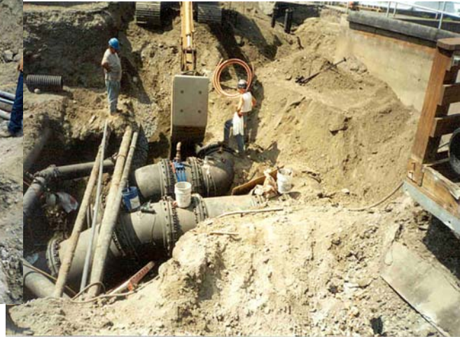
36-inch Diameter Pipe Crossing Existing Utilities
