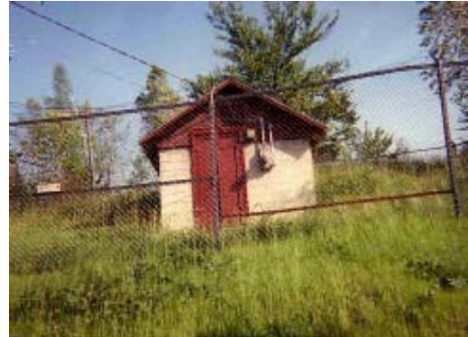
Booster Station in Beecher Falls, VT
