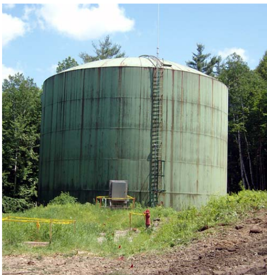
Former Steel Water Storage Tank
