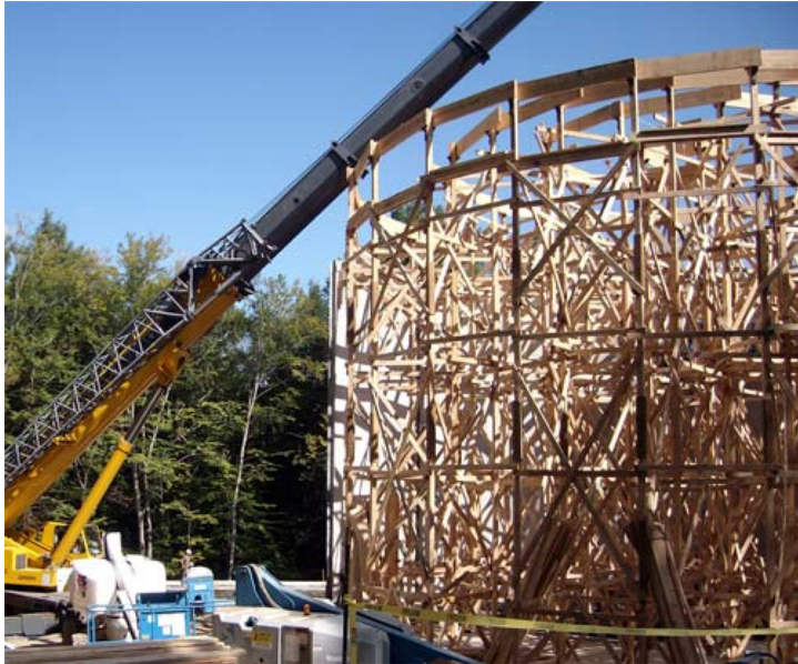
Interior Forming for the New Precast-Prestressed Concrete Storage Tank
