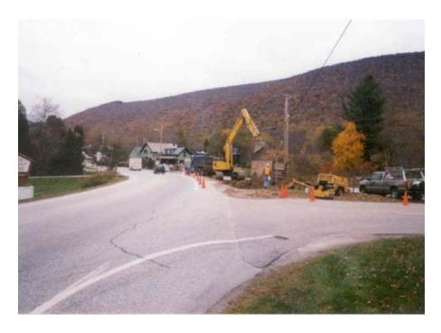
The Town of Manchester, Vermont in conjunction with a local developer extended the water system distribution main and the water system service area to allow a private school to be constructed and service extended to three motels. The 3,900 linear feet of 12-inch ductile iron pipe was installed along heavily traveled US Route 11/30 at the base of Bromley Mountain.
