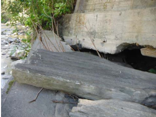
Damaged abutment
