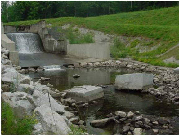
Lower Orange Reservoir spillway before the May 2011 storm
