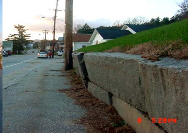
Reset Existing Stonework
