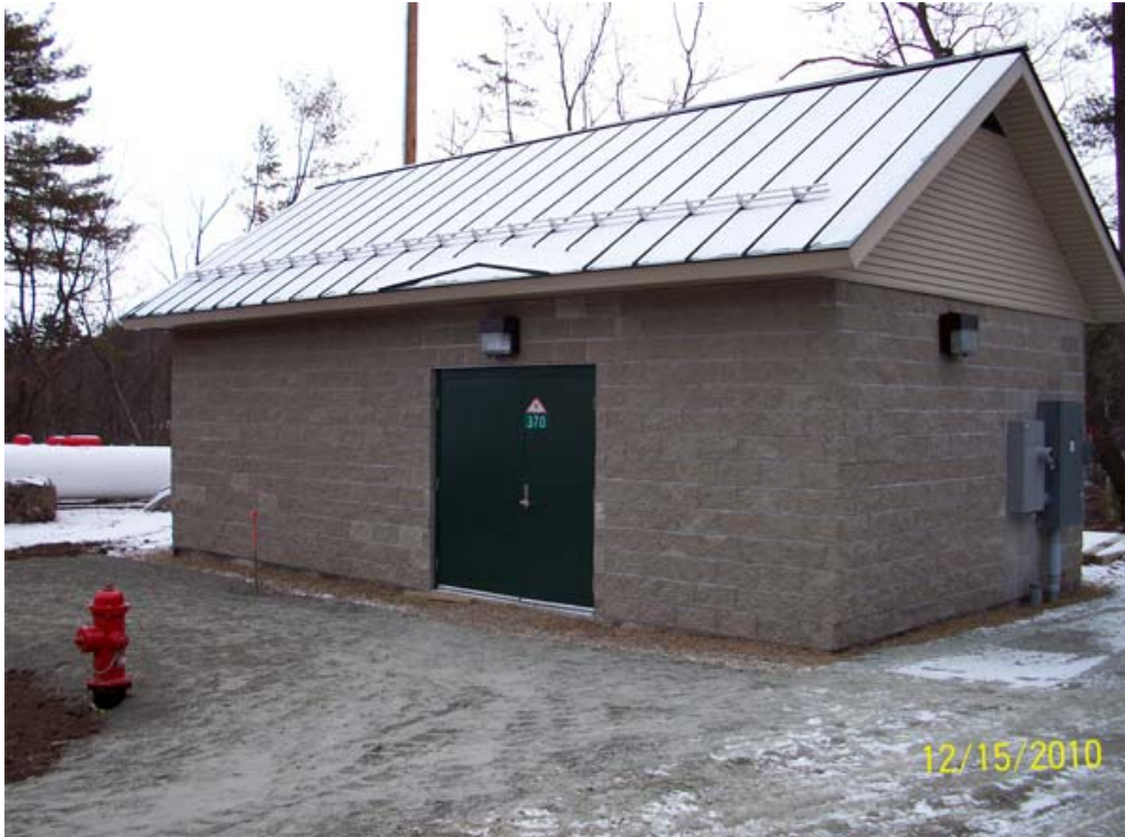
Exterior View of the Commonwealth Pump Station
