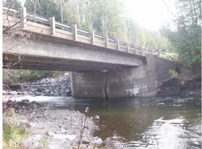
**Damaged Structure, Note Abutment in River**
