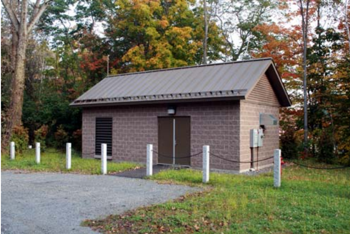
Exterior View of the New Bible Hill Pump Station
