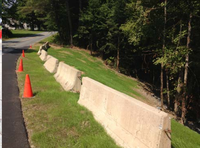
Stabilized bank pending permanent repairs
