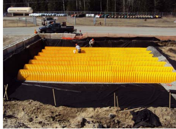
Infiltration Chamber Installation
