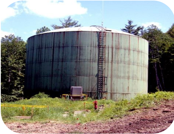
Former Steel Water Storage Tank
