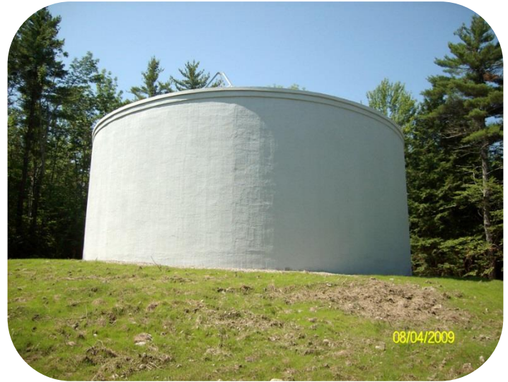
New Concrete Storage Tank in Place
