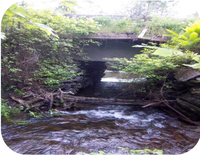
Existing Laid Up Stone Culvert
