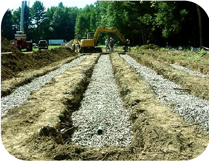
Typical Absorption Trench Disposal Field Prior to Backfill
