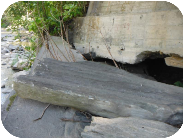
Damaged Abutment
