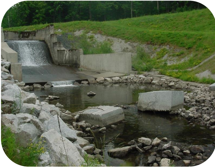
Lower Orange Reservoir Spillway Before the May 2011 Storm
