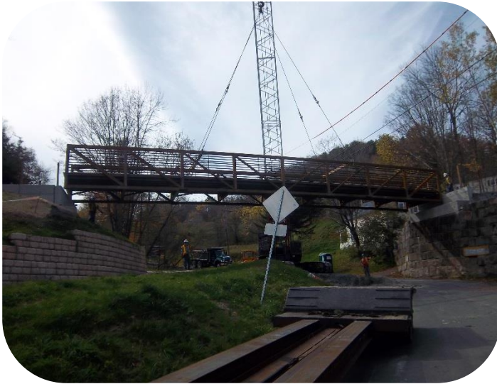
Lamoille Valley Rail Trail – Bridge #13 St. Johnsbury, Vermont
