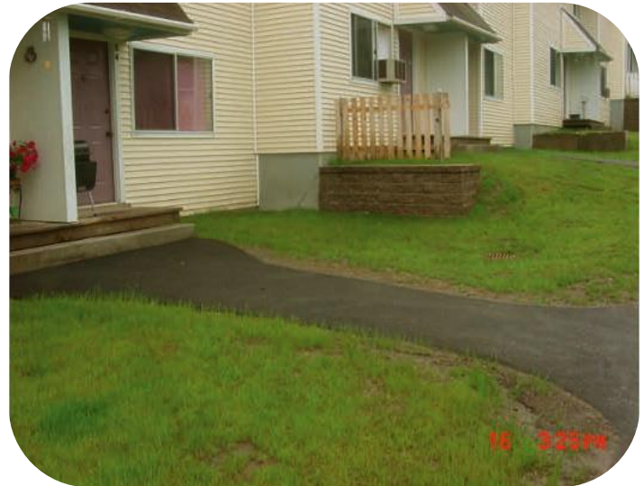
New Retaining Wall
