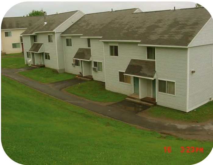
Highgate Apartments, New Sidewalks & Site Grading
