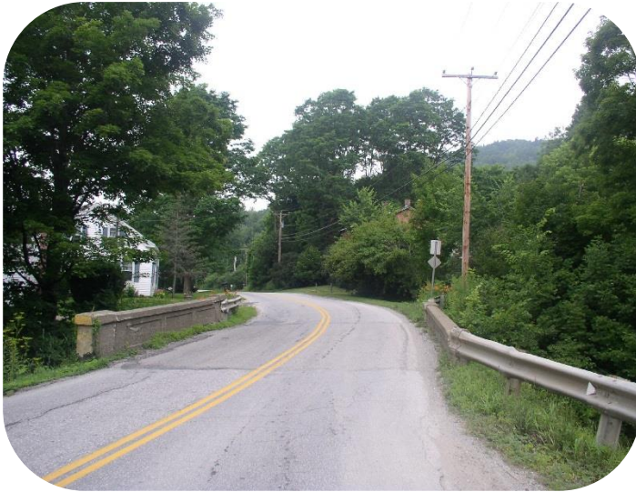
Town Highway Bridge No. 2, Poultny, VT
