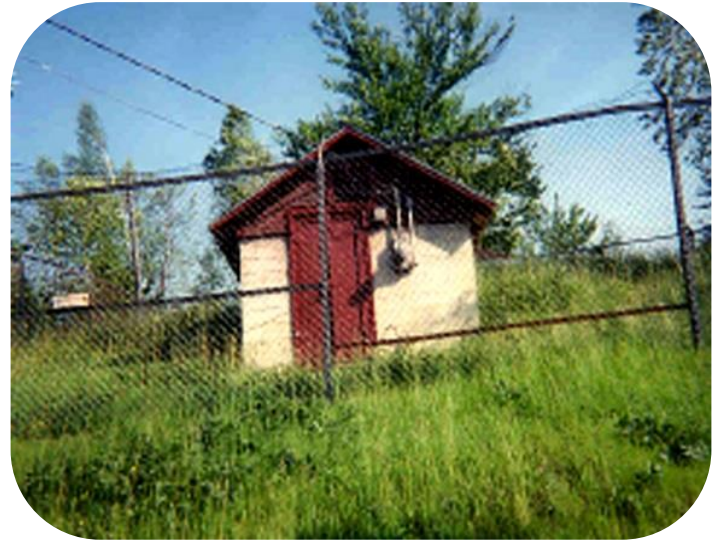
Booster Station in Beecher Falls, VT
