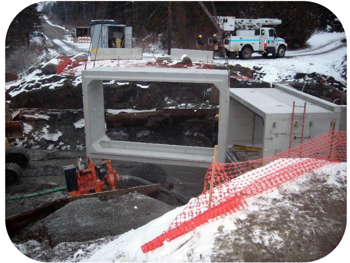
Construction Workers Set New 15-foot x 9-Foot Box Structure
