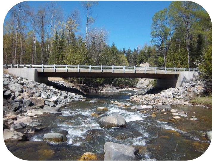
Completed Brownington Bridge
