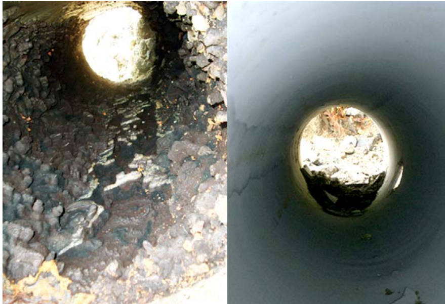
Water main before and after cleaning and lining activities.
