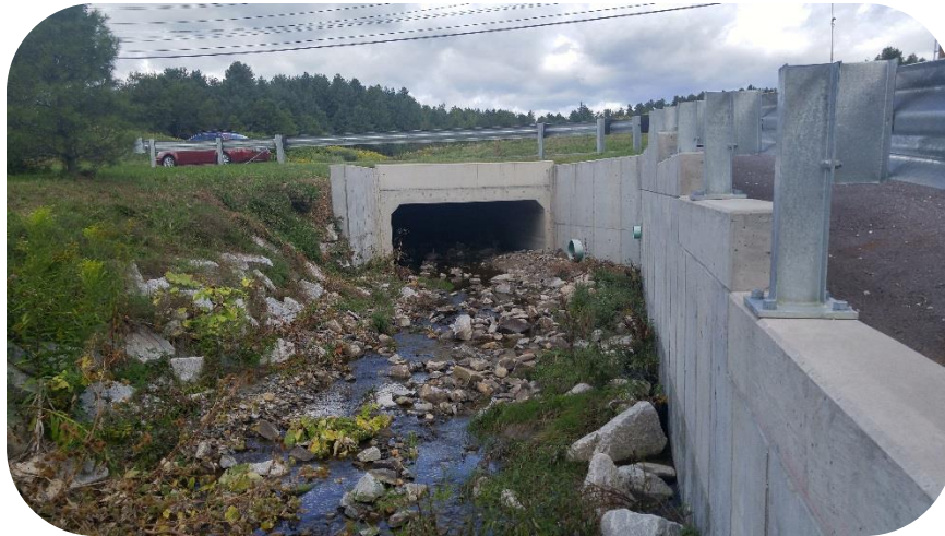
Culvert Outlet and Retaining Wall
