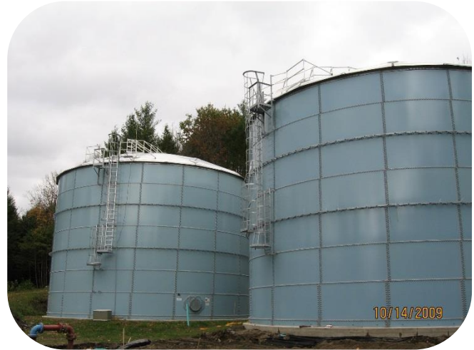
New Glass-Fused-to-Steel Tanks.
