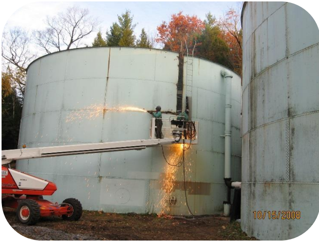
Crews Remove Old Bolted Steel Tanks Installed in 1932.
