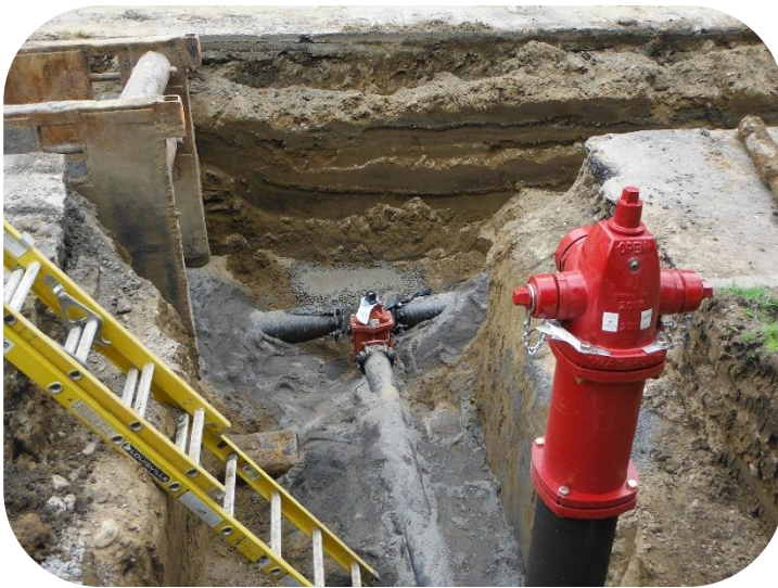
Hydrant Installation (School/Henry Project)
