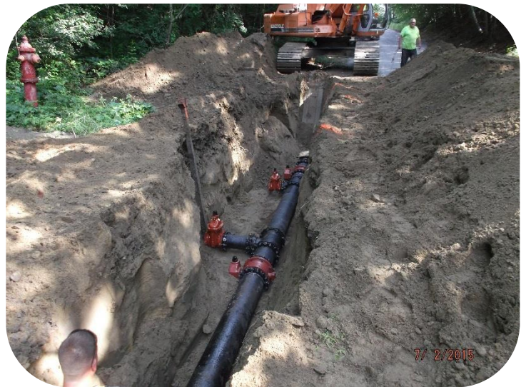
Water Main Installation on Industrial Drive (Route 5 North Project)
