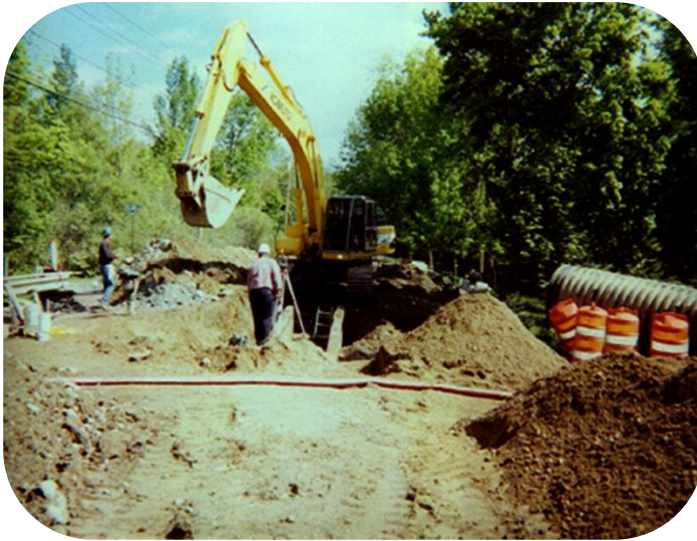
Engineer Checks Alignment of Major Intersection and Brook Crossing
