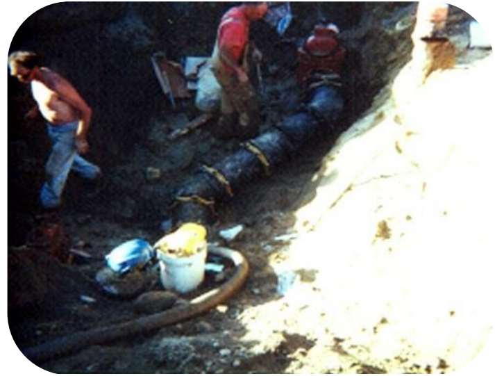
Contractor Installs Water Main Interconnection
