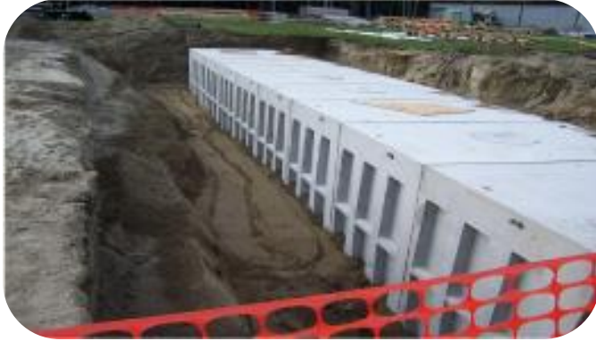
Stormwater Chamber Construction
