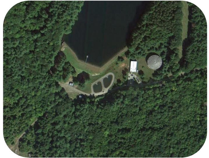
Aerial Photograph of Water Treatment Facility
