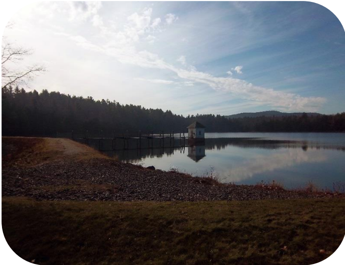
Gate House on Minard's Pond
