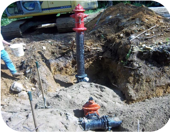
Construction in Progress
