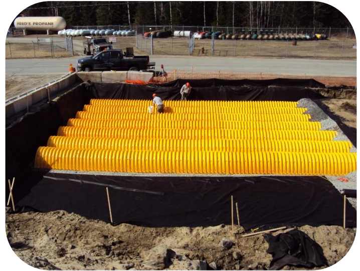
Infiltration chamber installation
