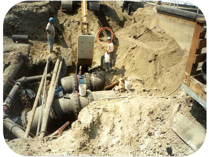
36-inch Diameter Pipe Crossing Existing Utilities
