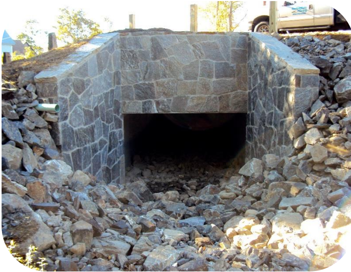
Stone Faced Culvert
