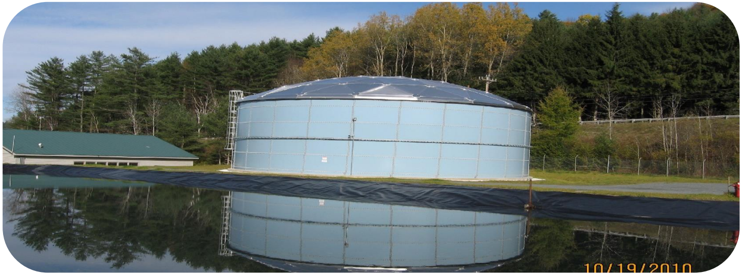
0.5 MG Clearwell at the Stiles Pond Water Treatment Facility
