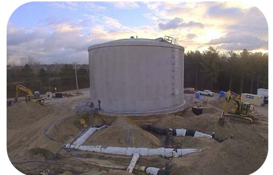
Construction of 30-inch and 36-inch yard piping
