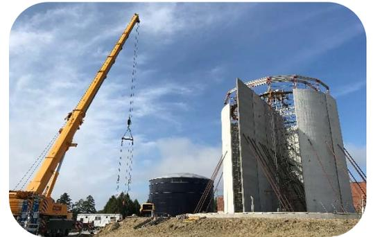
Construction of the 1 million gallon filtered water storage tank (interior baffle walls shown)
