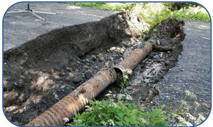
*Failed culvert in Barnet, Vermont after Spring 2017 storm event*
