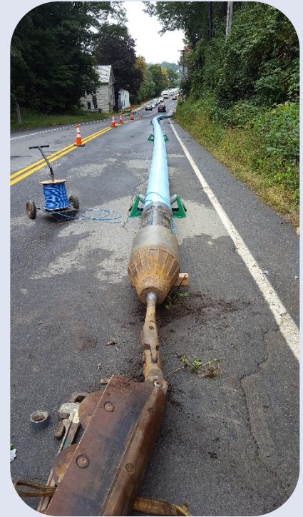
New Fusible PVC Pipe and Bursting Equipment
